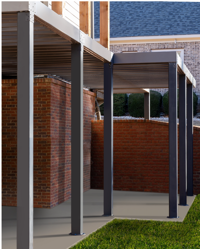
Figure 1: New Castle Steel exterior deck with 12 ft. tall support posts
